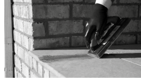
PIC 1. Fill joint with grout.
