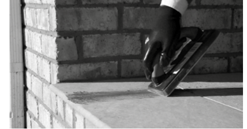
PIC 2. Remove excess grout with clean water.
