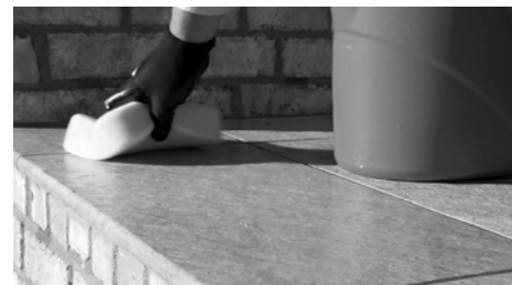
PIC 5. Removal of excess grout residues with hard brush.
